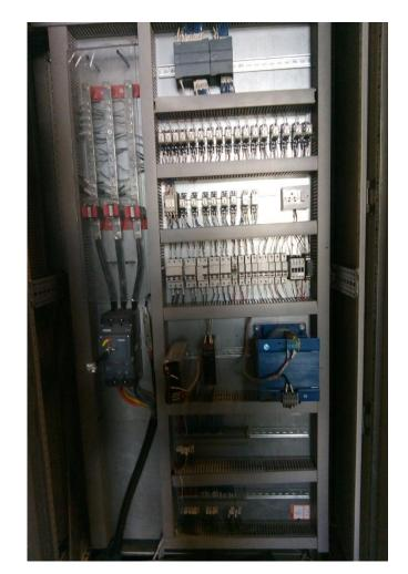
Figure 3.1 :Control panel picture PLC side
