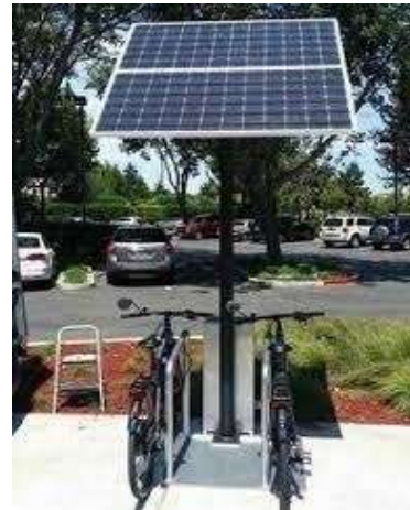
Figure 3 : Solar powered E-cycle charging station
